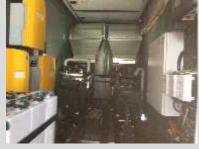
Diesel Generator Two units synchronized 33 kW diesel generators are consist of Perkins engine and Stamford alternator to provide continuous power no matter what.
