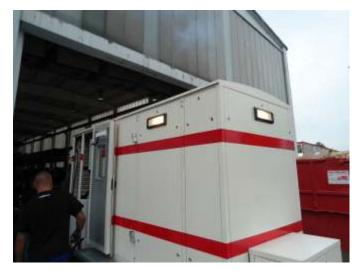
At Kunz we are testing our generators at a supplemental load of 25% of nameplate rating for 30 minutes, followed by 50% of nameplate rating for 30 minutes, followed by 75% of nameplate rating for 60 minutes, for a total of two continuous hours. Furthermore, KUNZ tests its sets by dummy loads again running at 100% of the rated power capacity for 15 minutes.
