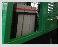
**Batteries** 24 units, each 2 V batteries, are providing 910 Ah and 2000 A with highest longevity and cycle stability. It saves the sun or daytime energy to provide enough power at night time.
